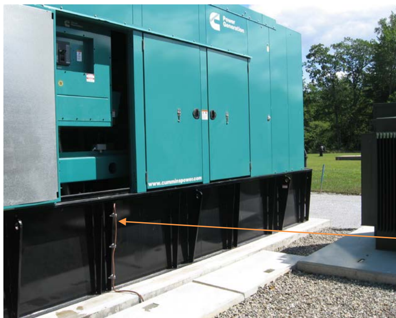
Connection to grounding electrode system
